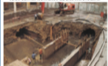
View of the canal construction site in Modena
